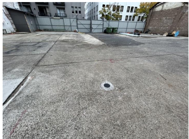
Figure 18 - View north detailing a ground monitoring well.
