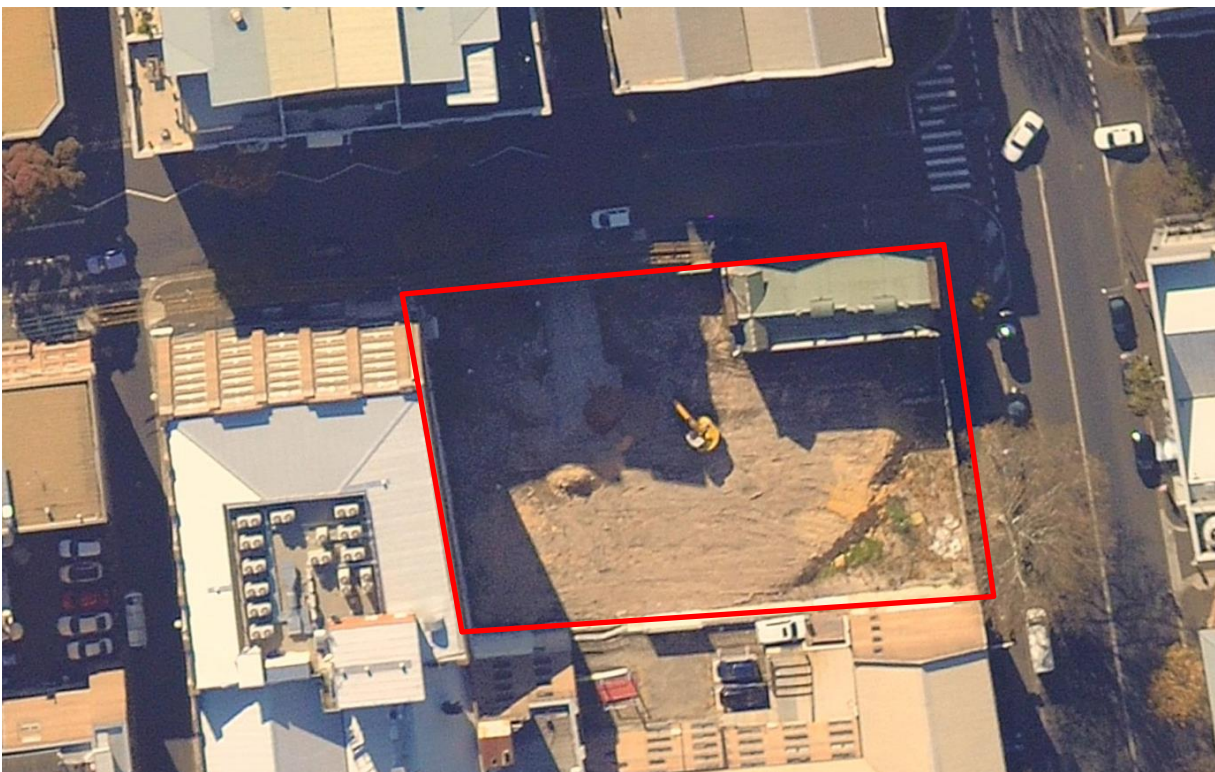
Figure 14 - Aerial photograph 2010 following demolition of previous structures within the subject area and addition of fill layer.
